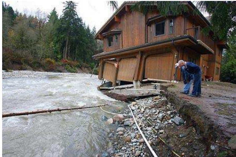
Figure 4. House destroyed due to channel migration along the Raging River.
